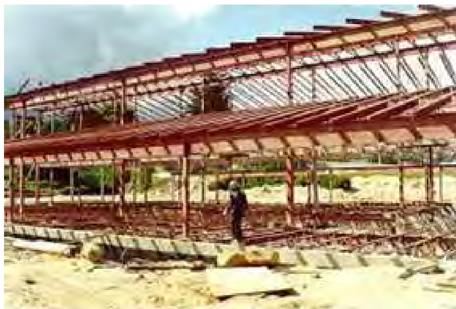
Figur A. 10 Roy Stibbs Elementary School, Kanada
